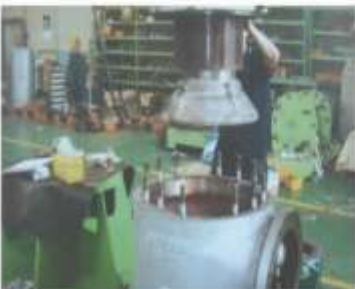
Maintenance for Safety Valve
