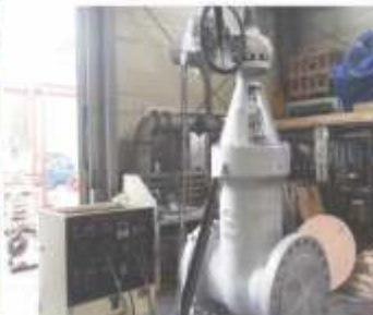
Maintenance for MOV Gate Valve
