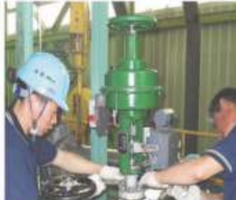
Field Work for Control Valve
