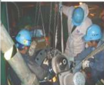
Field Work for Main Feed Water Valve
