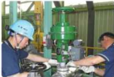
▶ FIELD WORK for CONTROL VALVE
