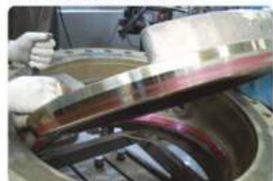
▶ Maintenance for Tilting Check Valve
