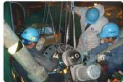
▶ FIELD WORK for MAIN FEED WATER VALVE
