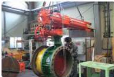
▶ Maintenance for Butterfly Valve
